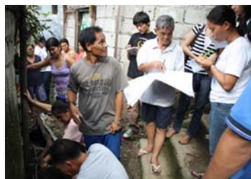
(Left) The walkway at the Creekside community being planned and built.
