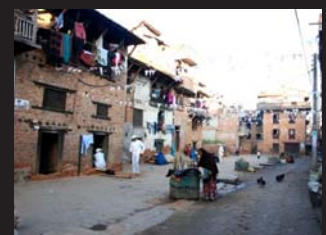
Another project improved the drains and laid new paving stones in this public square in the Kutujhol community.
