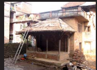
One project involved repairing the clay tile roof on this beautiful old public "phalcha" rest house in Laskuti.
