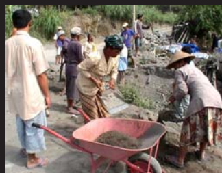
▲ Arkom's project in Mount Merapi started with the construction of temporary houses and latrines, then focussed on restoring water supply, and then on repairing roads like this one in the Kalitangah Lor Village.
