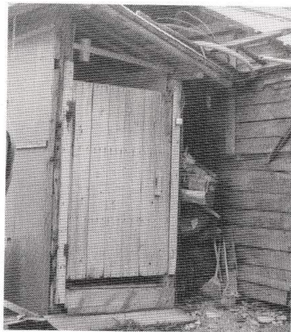
• Communal toilet: an outdoor toilet shared by several households.
