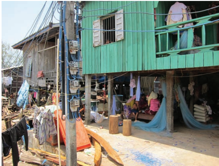
PHOTO 3 Street lighting and electricity meters in the Sansom Prak community in Khemara Phoumin, Koh Kong province, Cambodia
