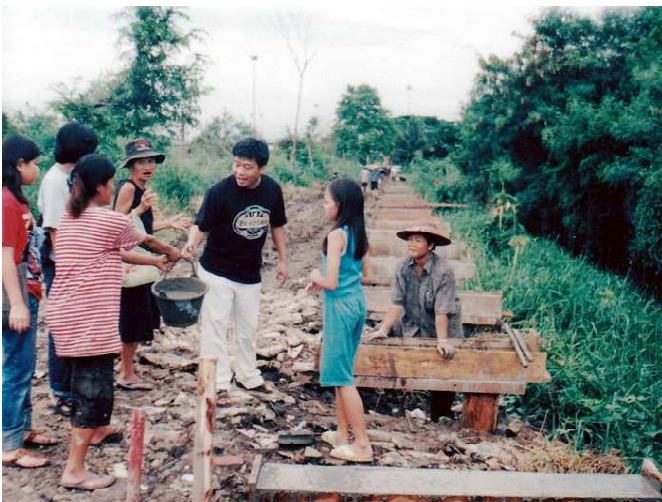
The concrete walkway was built on short columns along the edge of the drainage canal, and everyone in the community pitched in to help. The walkway allowed the people to come and go without getting their feet mucky, and made it possible to bring in construction materials easily.
