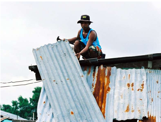
Most of the families in Klong Lumnoon were careful to preserve any building materials from their old houses which could be used in the new houses, to keep construction costs down: tin and fiber roofing sheets, timber, cement blocks, bricks, doors and windows).
