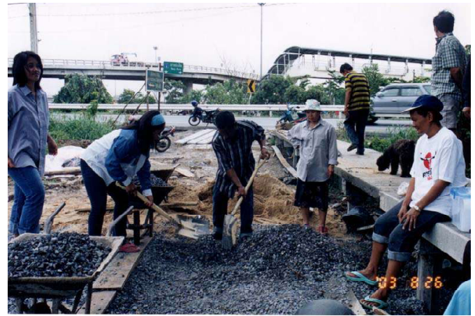
The first step in the community's physical transformation was the construction of a 520-meter concrete walkway into the community.
