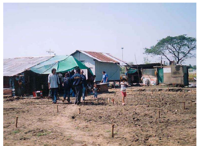
Once the 4,000 square meter site was filled, the people worked with the architects to peg out the house plots, to prepare for the house construction.
