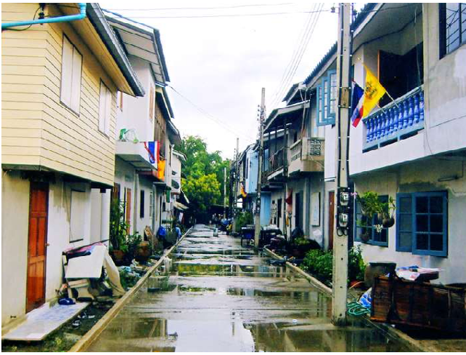
▲ A rainy day photo of one of the newly-finished lanes at Klong Lumnoon, with concrete paving, storm drains, electric poles and planting strips.
