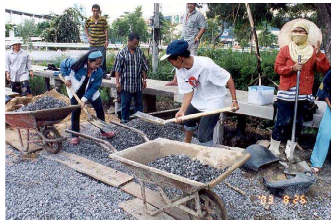
The concrete walkway was built on short columns along the edge of the drainage canal, and everyone in the community pitched in to help. The walkway allowed the people to come and go without getting their feet mucky, and made it possible to bring in construction materials easily.
