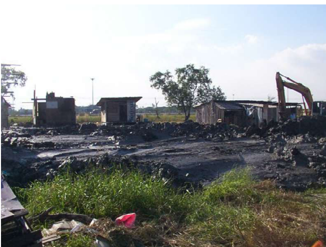
After the site had been cleared, the next step was to have a meter of dense, clay soil trucked in, to raise the land above flood levels.
