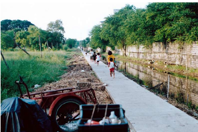
When the raised concrete walkway was finished, one community leader commented, "I'm glad the walkway is done and I'm proud of it. But I'm sorry that a project that brought us all to work together so well is over."
