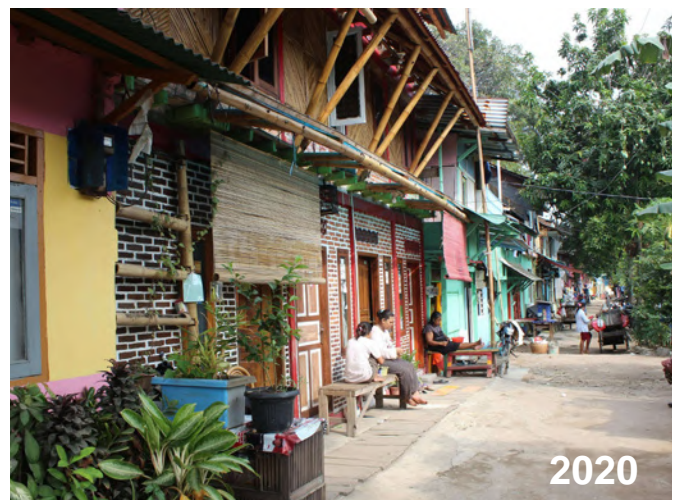
▲ These two photos illustrate the before and after conditions of the prototype houses. The initial state, characterized by a patchwork of old materials and a narrow road, transformed into a stable, colorful home with higher ceilings, better ventilation, and proper road, drainage, and sanitation facilities.
