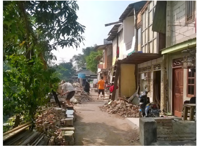
▲ The facades were carefully demolished with the goal of salvaging as many materials as possible for reuse in the renovation.
