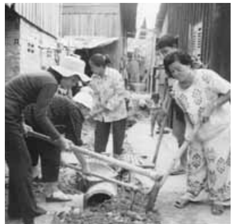
Comprehensive upgrading at Ros Reay : People worked around the clock to dig the trenches and lay the pipes for their new underground sewer and storm drainage system, just part of their upgrading plans.
