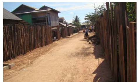
AFTER : This is the same road, after the underground storm drains have been laid and the road resurfaced.
