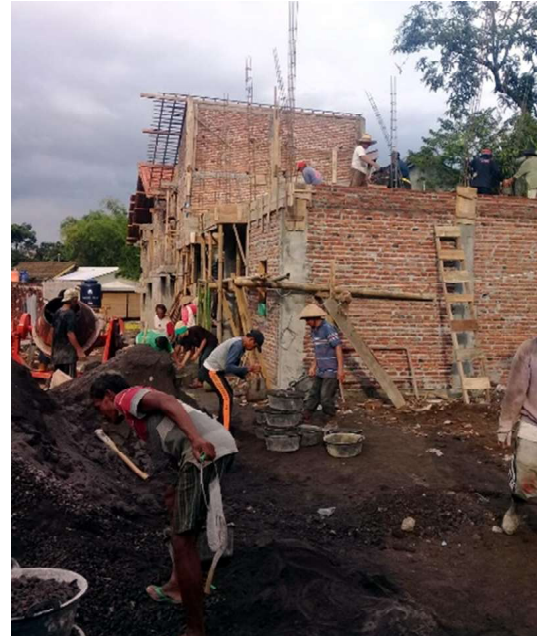
▲ Excavating for the concrete pile foundations of the new houses (above) and helping out on the site as the walls are going up (right).
