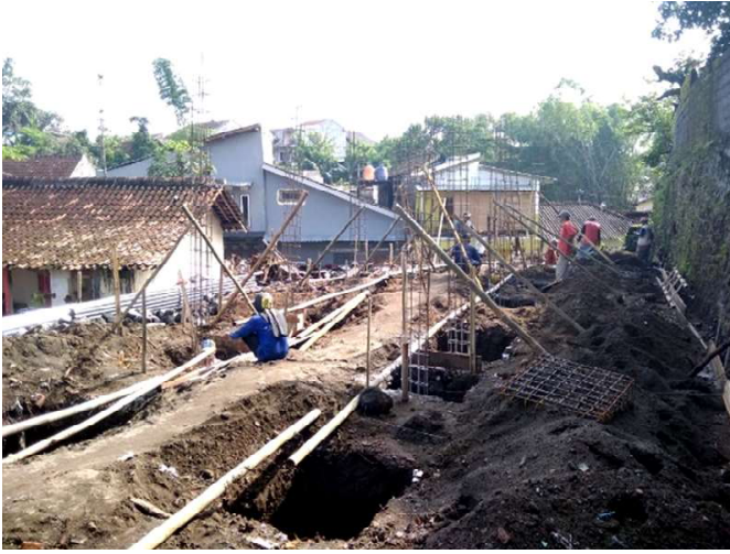
▲ Excavating for the concrete pile foundations of the new houses (above) and helping out on the site as the walls are going up (right).
