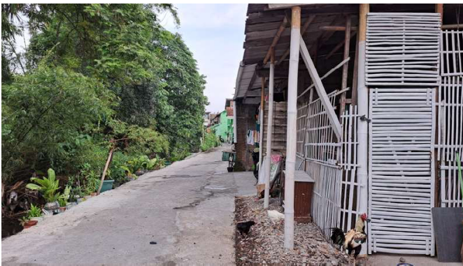
▲ A photo taken during the work of upgrading the river-fronting houses, which have been chopped off to make way for the 3-meter inspection road.
