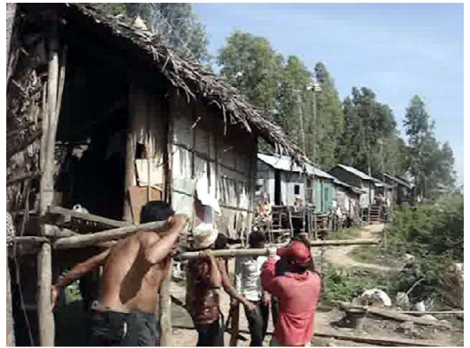
To clear the site for construction, they actually moved the old houses to nearby land, so people would have somewhere to stay during the construction.
