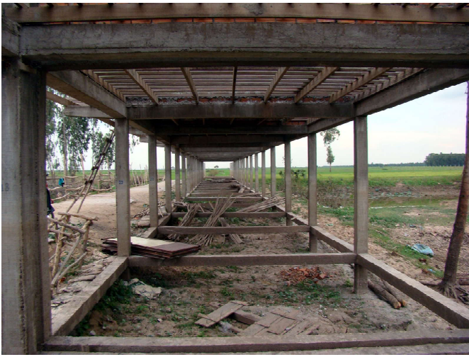
Because the budget was so tight, the houses were left unfinished down below, with the idea that people could live upstairs, and then finish the downstairs as they could afford to do so.
