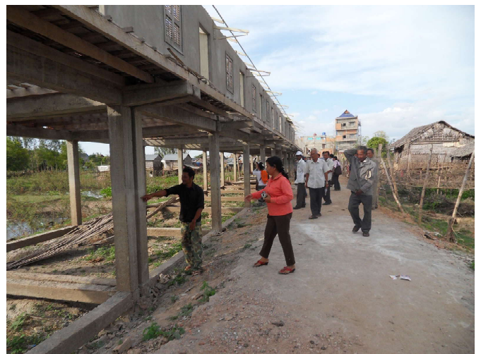
A little later in the construction process, with the community construction management committee negotiating with the skilled masons.
