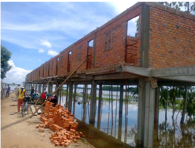
The construction was slowed down a bit by heavy flooding from the Mekong River, but not stopped. The Khmers are used to living with water.
