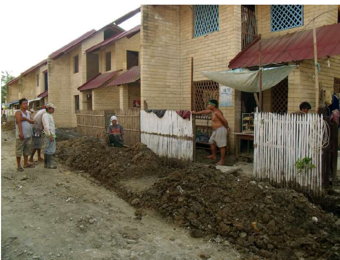
The work on the storm drains, with covered channels that are 2.5 meters deep (right), started in one section of the RVHOA project where people had already moved in.
