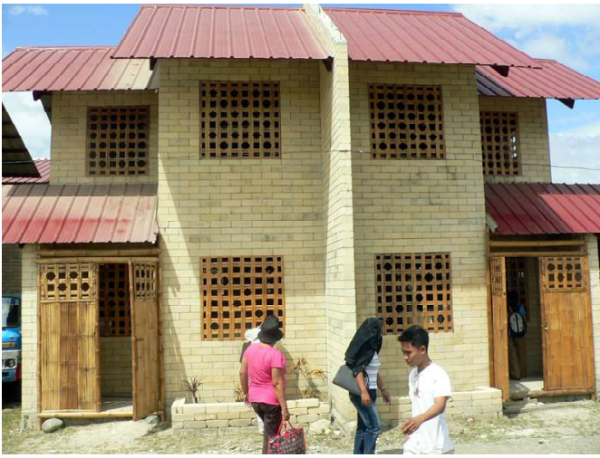
In these two demonstration houses, some inexpensive bamboo doors, stairs and window grilles are showing people one option for finishing the house enough to move in.
