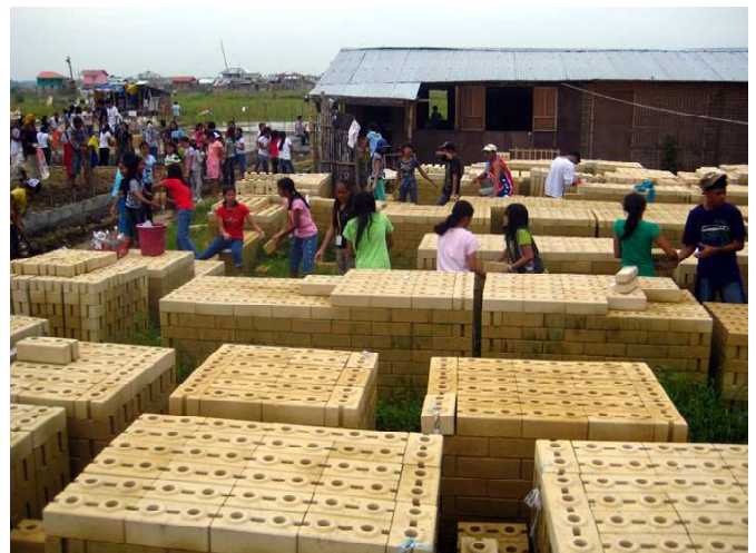
The big task of moving all those ICEB blocks from the block-making area to the building site was helped by lots of good-natured volunteers.
