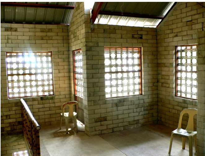
A shot of the upstairs room, with plywood floors and a softly dappled daylight coming in through the bamboo window grilles.
