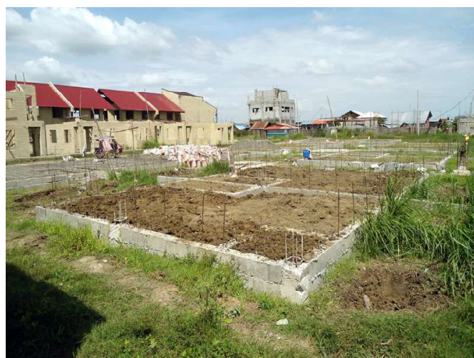
▲ A cheerful group of community workers helping dig the trenches for the foundations of one block of new houses at RVHOA. And (above right) a foundation ready for the ICEB block walls.
