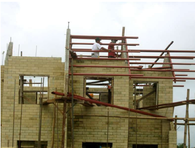
▲ A group of houses that are close to being finished, with the steel roofing purlins being put in place, and the galvanized steel roofing sheets being unloaded from the truck.
