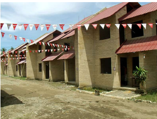
▲ To keep them affordable, the houses were left partly unfinished, and it was up to people to add the doors, windows and other finishes.
