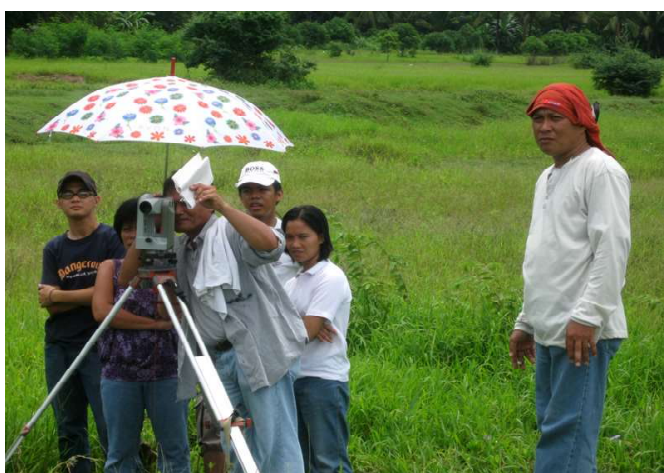
Once the subdivision plan was approved by the city, the architects and engineers surveyed the site, to mark out the house plots and roads, with assistance from students from nearby technical colleges
