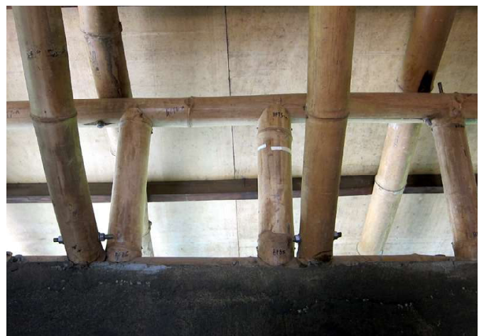
The bamboo houses are very carefully crafted, with every bamboo pole being numbered and bolted in place, and lots of beautiful details.
