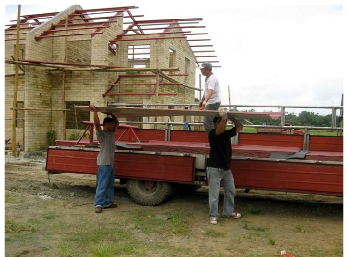
▲ A group of houses that are close to being finished, with the steel roofing purlins being put in place, and the galvanized steel roofing sheets being unloaded from the truck.
