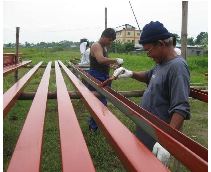
▲ Community members paint rust-resisting red-oxide paint on the steel purlins that will hold up the roofing sheets on a group of houses.
