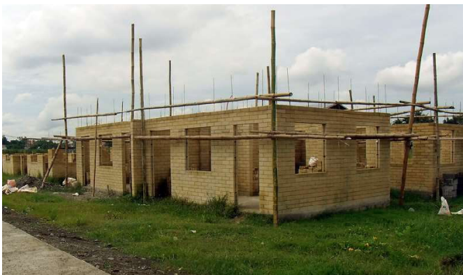
▲ Photos from various stages of the construction of the ICEB houses in RVHOA. It took about four years to complete all the houses.
