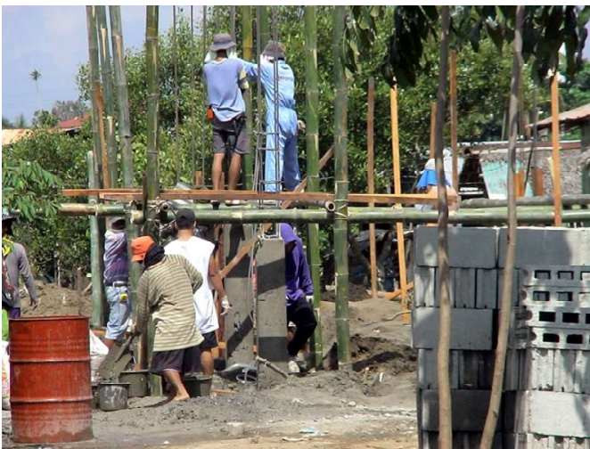
More photos from the construction of the row houses, with bamboo scaffolding put up for the concrete columns. With so many helpers on the site, the construction went very quickly.
