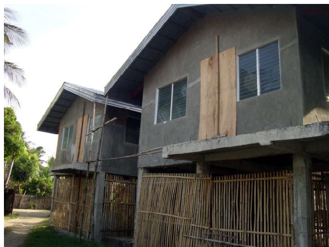
Here are two of the detached single houses, right after being built (above left), and a few months later (above right), when the residents had begun to put in some aluminum louvered windows and plaster the outside. Later, they would enclose the ground floor rooms.
