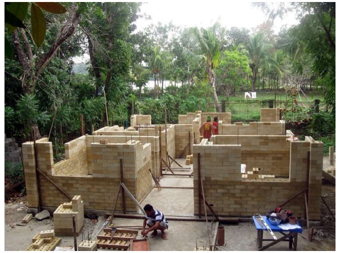
The soil of Iloilo turns out to be very well-suited for making ICEB blocks and produces a honey-colored block that doesn't have to be painted.
