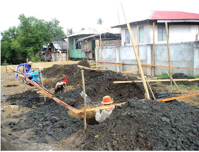
Work began with the construction of the ten row houses. In the photos above, the holes for the foundation and reinforced concrete footings are being dug by community members.
