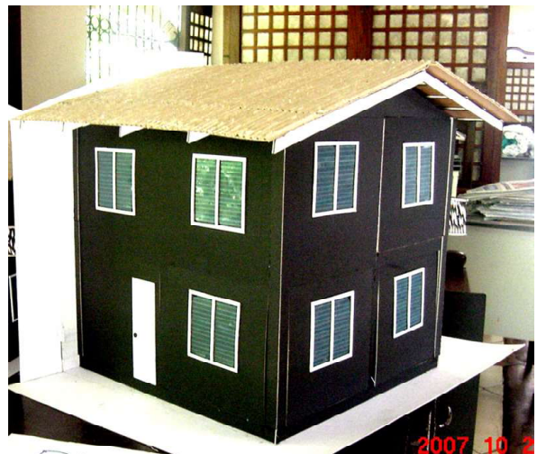
Here are models of two types of the detached single houses, which could be built within the CLIFF loan limits, if the lower floors were left unfinished. All the detached houses were designed to be built right on the property line, with fire walls, to save space for future additions.
