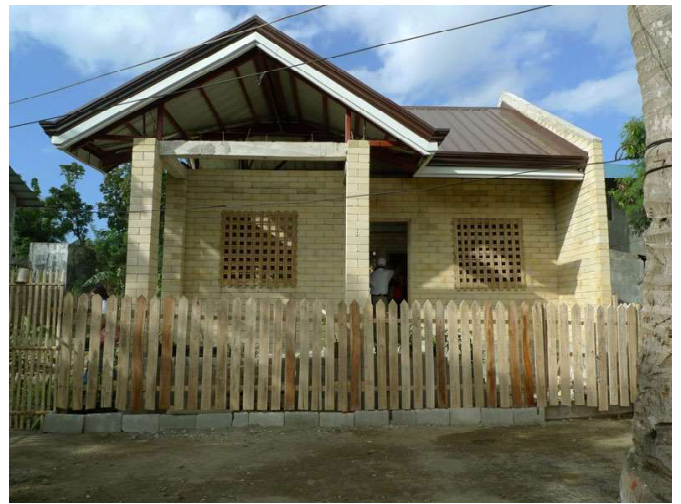
More photos from the construction of the ICEB block demonstration house in Kabalaka. To keep costs within the CLIFF loan limit, there wasn't enough budget for fancy doors and windows, so they used simple bamboo initially.
