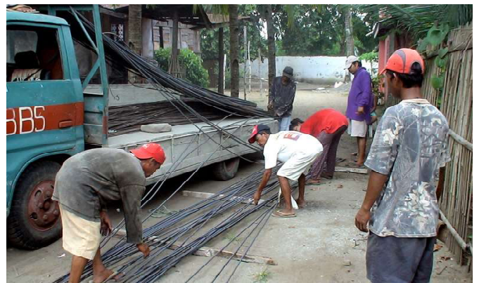
A truckload of steel bars being unloaded at the entrance to the Kabalaka community, with community members keeping tabs.
