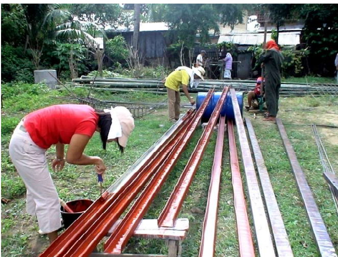
Here community members are painting the steel purlins that will be used in the roofs of the row houses with rust-resisting red oxide paint.
