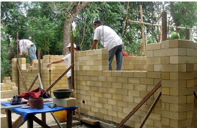
The ICEB block demonstration house in Kabalaka was another first for Iloilo, so the construction became a training course for everyone.
