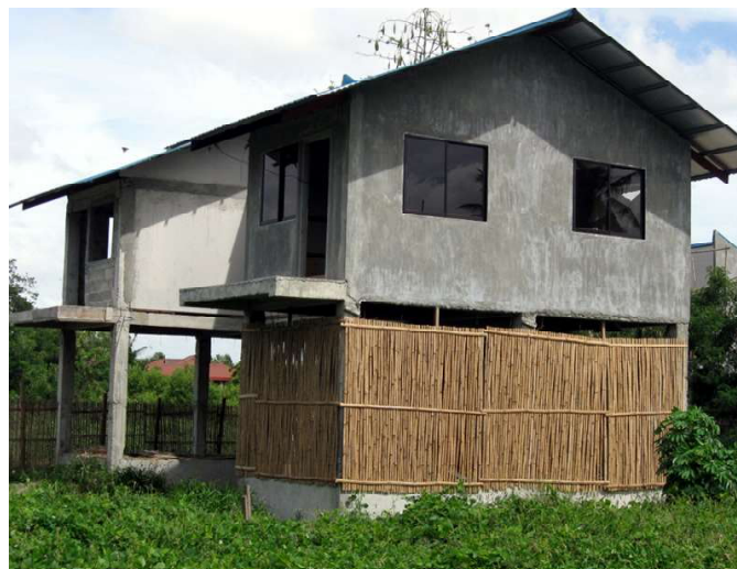
Here are two more detached single houses, which used another design, towards the end of the construction process.
