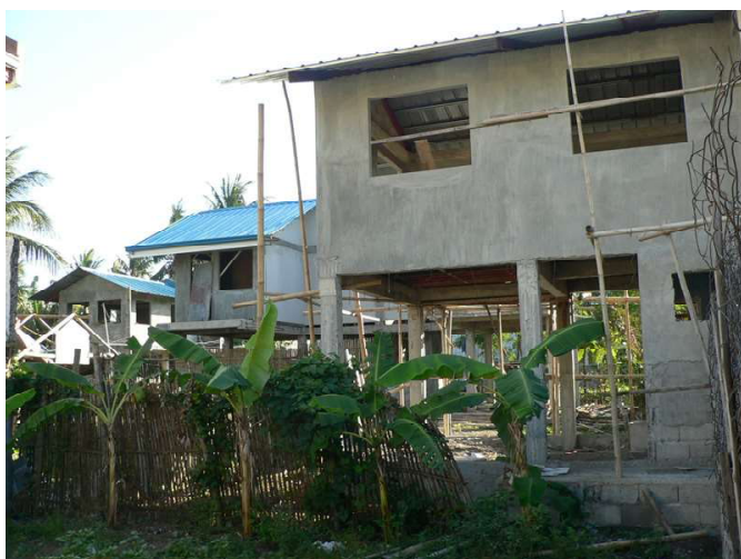
A photo taken on the Kabalaka site in April 2009, when the construction of the 21 houses in the pilot project was coming to an end.
