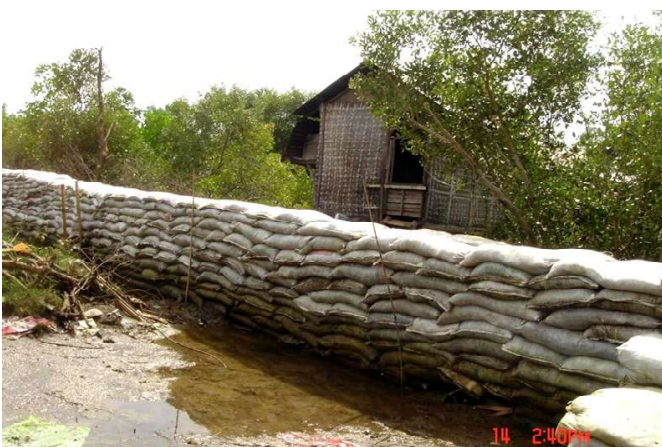
This is what the work looked like after the sand bags and bamboo rafts had been stacked up to one meter above flood level. Next, soil was banked up on both side of the sand bags.
