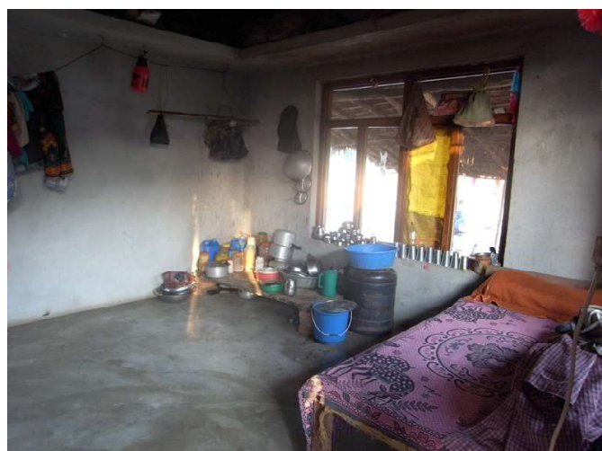
A light-filled room in one of the upgraded brick houses, with a paved concrete floor, and high shelves for storing things used less often.
