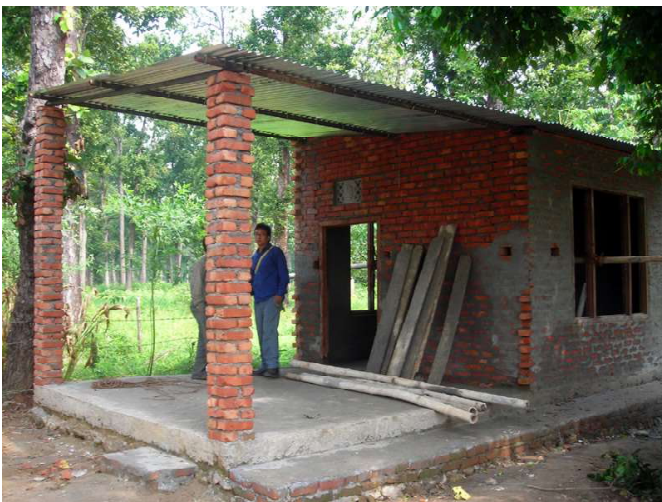
The houses were all different, but all of them used the simplest building systems and the most readily accessible local materials like brick, fiber cement roofing and timber. The timber for much of the project was provided by the Forest Department at subsidized rates.
