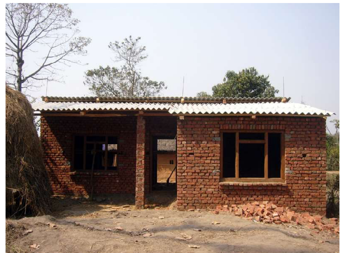
The houses were all different, but all of them used the simplest building systems and the most readily accessible local materials like brick, fiber cement roofing and timber. The timber for much of the project was provided by the Forest Department at subsidized rates.
