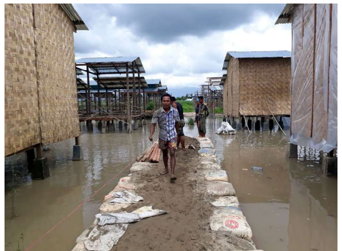
▲ Sandbags were used to define the boundaries of the raised main roads in the settlement, and the space in between was filled in with soil and sand to reach above-flood levels and allow people to move around the site and build their houses.
