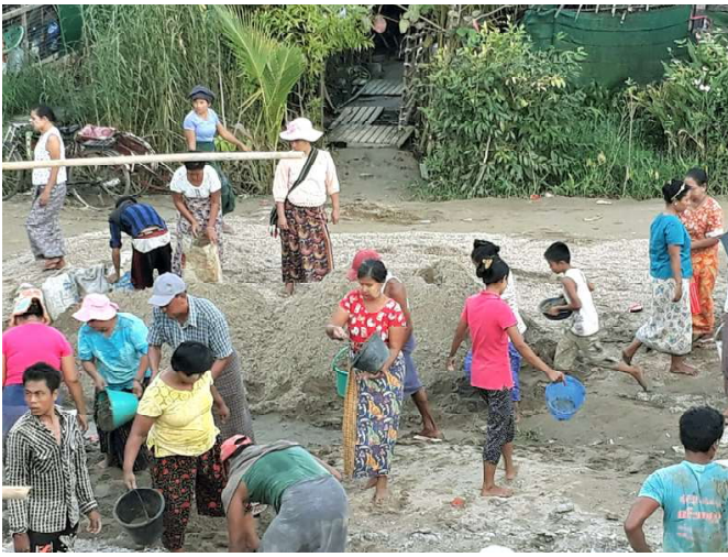
▲ The community center at Taw Win was built in just five days, with lots of friends from other savings groups and collective housing projects coming every day to carry materials, mix concrete and help with the construction.
