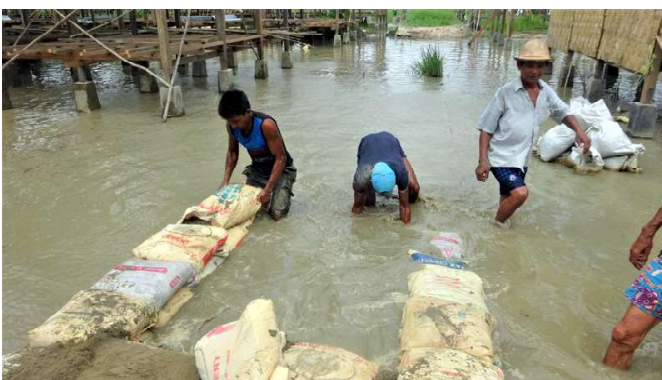
▲ Sandbags were used to define the boundaries of the raised main roads in the settlement, and the space in between was filled in with soil and sand to reach above-flood levels and allow people to move around the site and build their houses.
