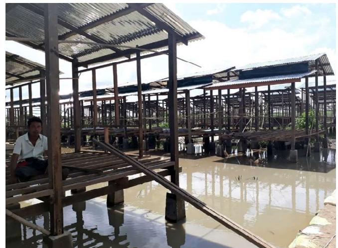
▲ Construction started during the monsoon season, and the land soon flooded, making it extra difficult to clear the land and lay the foundations for the houses. A team of carpenters familiar with the women’s network built the structural parts of the houses and the residents did much of the simpler tasks, with help from the carpenters.
