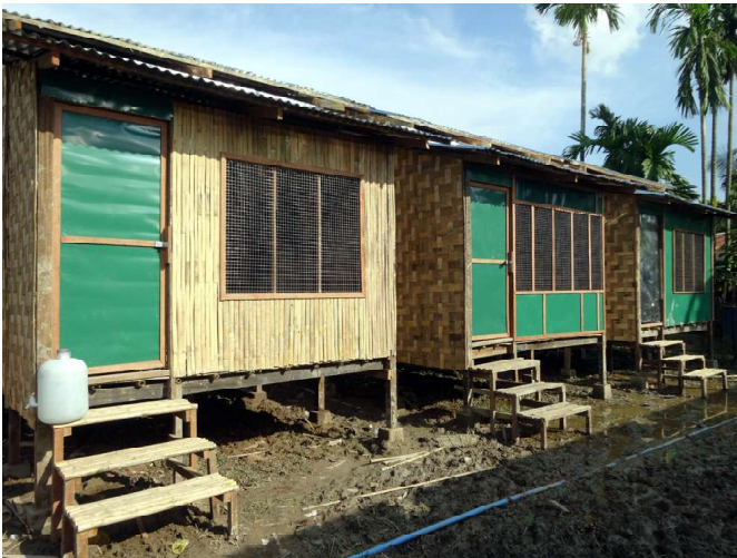
A row of three of the finished houses ready for the families to move in.
