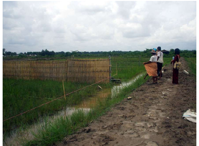
▲ Putting up some fencing and stakes to mark the boundaries of the land the women had purchased, in preparation for construction.
