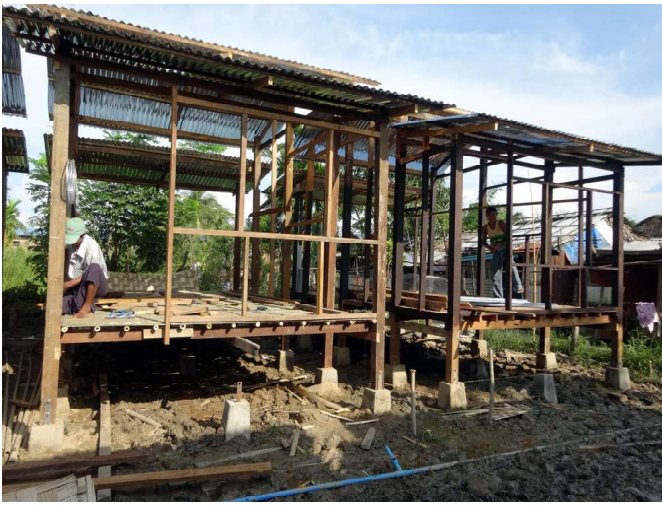
Two of the new houses with the frames and roof complete, and almost ready for the windows and siding to be put on.
