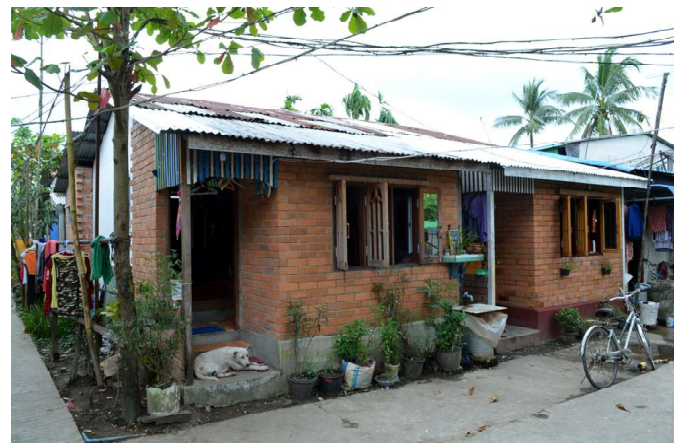
▲ Here are two front-row houses that have been upgraded from wood to brick and concrete. There will be many more of these kinds of upgrades as the families' capacity to invest in their houses increases.
