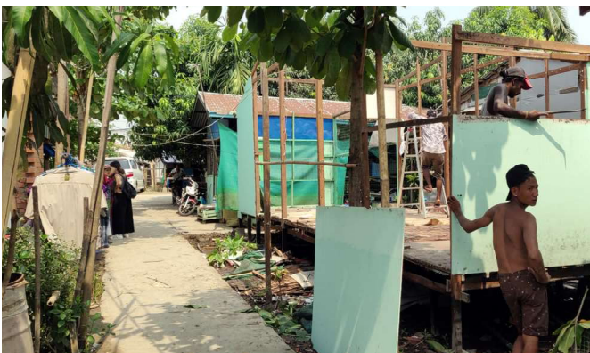
▲ Here is one house that is being dismantled before the house was totally rebuilt in bricks and concrete (right) - the community's first such upgraded house.
