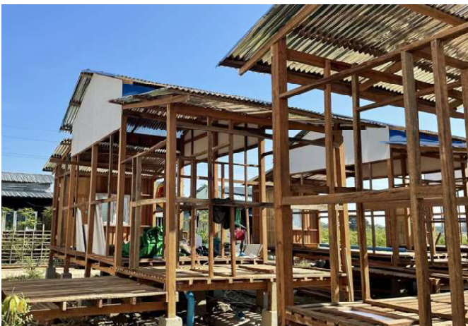
▲ Corrugated tin sheets were added for the roof, and fiber-cement boards were used for very light walls. The front wall of each house was built with more expensive timber planks, so the houses would present a more dignified face to the street.
