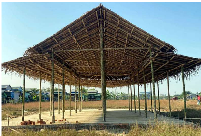
Recently, the community built this open-air thatch and bamboo market where people can sell their vegetables and community products.
