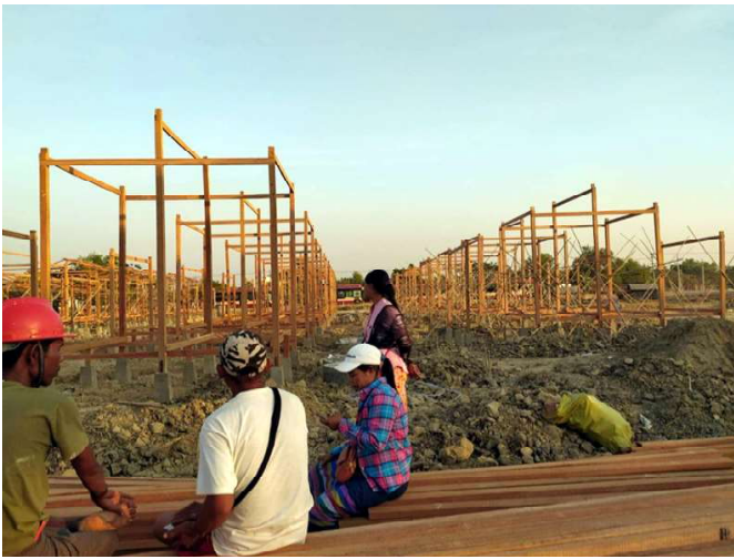
▲ The process of constructing the houses went very quickly and was quite systematic, thanks to the experienced carpenters who had accumulated a lot of experience building the earlier community-led housing projects. After the concrete footings were arranged on the site, the wooden structure came next.
