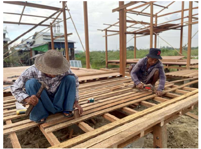
▲ The process of constructing the houses went very quickly and was quite systematic, thanks to the experienced carpenters who had accumulated a lot of experience building the earlier community-led housing projects. After the concrete footings were arranged on the site, the wooden structure came next.
