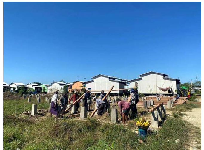
▲ Corrugated tin sheets were added for the roof, and fiber-cement boards were used for very light walls. The front wall of each house was built with more expensive timber planks, so the houses would present a more dignified face to the street.
