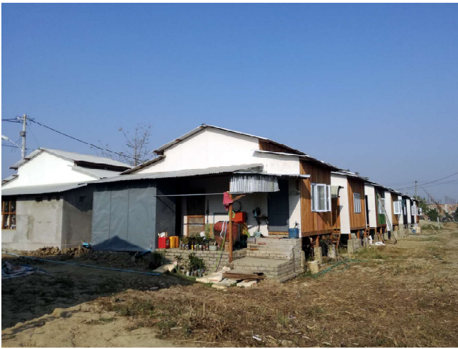
▲ Within a few weeks of moving in, people started constructing additional rooms on the side and painting the facades of their new houses.
