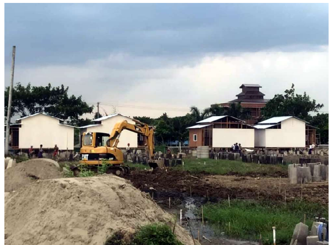
▲ To speed things up, the land filling continued on parts of the site at the same time the houses were being built on other parts of the site.
