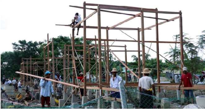
▲ One of the best ways to keep the cost of the houses as low as possible was to use inexpensive local materials and simple building systems and techniques that everyone understands and can build, without any special training or gadgetry.
