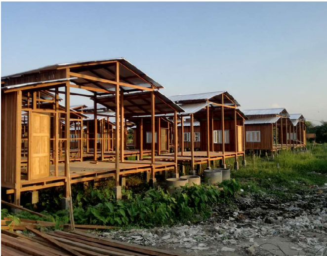
▲ In this photo of a group of partly finished houses, you can see the soak-pit tanks where the toilets behind the houses will drain.
