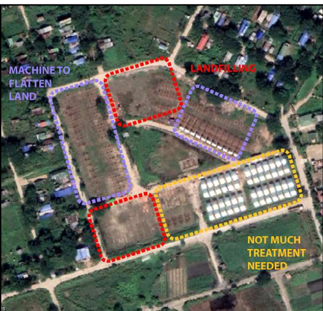
▲ This map shows the parts of the site that had to be filled with 1 - 2 meters of fill to bring them up to above flood level (red), and the other parts that were OK and just needed to be levelled (yellow and purple).
