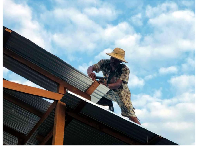
▲ Galvanized iron roofing sheets being fixed to the light roof structure. Nobody will claim these are 100-year houses, but they're good enough for now, and people can upgrade them later on.
