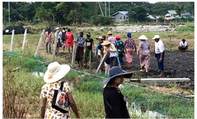
▲ Another photo from the days of clearing the new land and marking the boundaries of the individual house plots, with the staff of the local government.
