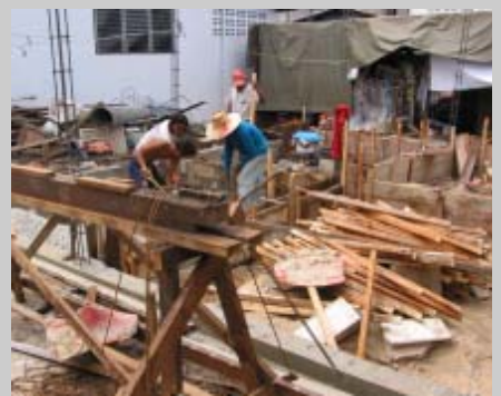
To stretch their infrastructure subsidy, the people are doing all the work themselves.
