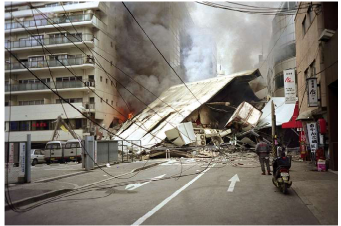
▲ The great earthquake that hit Kobe on January 17, 1995, killed 4,600 people in the city. Here the Hanshin Expressway, at the north of Mano District, has collapsed.
