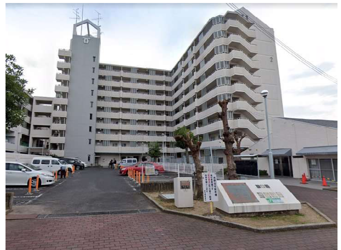
6 This municipal block of flats provides subsidized public rental housing to 107 households, including those whose houses were on the site before.
