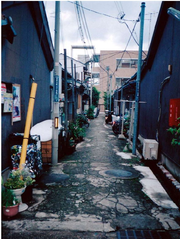
▲ Some of Mano's small inner lanes have been left more-less as before, but with much improved drainage, paving and infrastructure.
