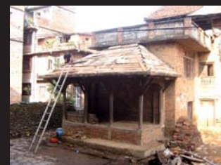
One project involved repairing the clay tile roof on this beautiful old public "phalcha" rest house in Laskuti.
