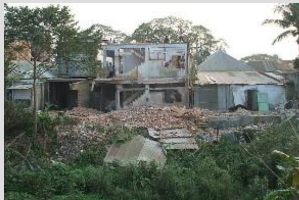
Part of buildings on setback being demolished in Manikganj city as part of the interim government’s eviction drive
