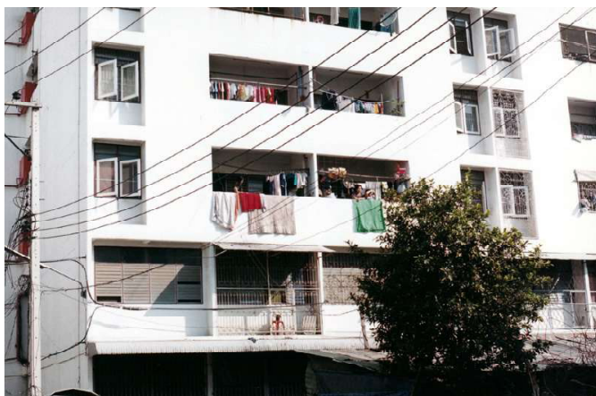
The apartments are all entered from open corridors which surround internal courtyards. And all the units have generous balconies on the outside, with space for drying laundry and making for good cross-ventilation.
