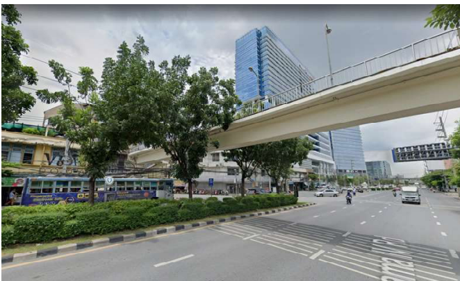
▲ Here is a photo of what the Rama IV Road looks like today, in 2021, in the stretch that runs in front of the former Thep Prathan community (on the left).
