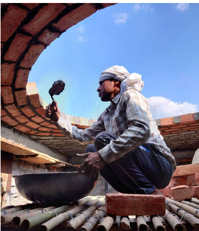
Here the arched walkways that will connect all the buildings are being constructed by the local contractor's masons on the site.
