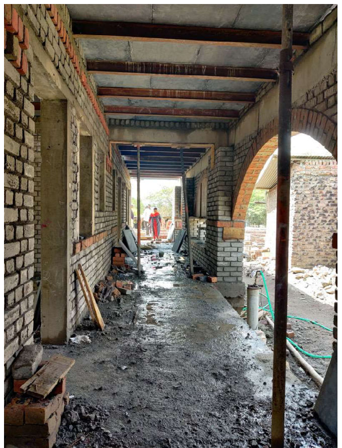
More photos from the construction of Building number 6, taken in September and October 2020. The black-cotton soil conditions on the site meant that the pile foundations had to go down five meters, so the foundations accounted for nearly 30% of the construction costs.
