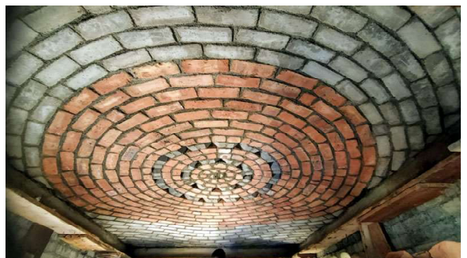
To save on steel and cement, the 3rd-floor rooms are all spanned with these beautiful shallow domes, which support the roof terraces.
