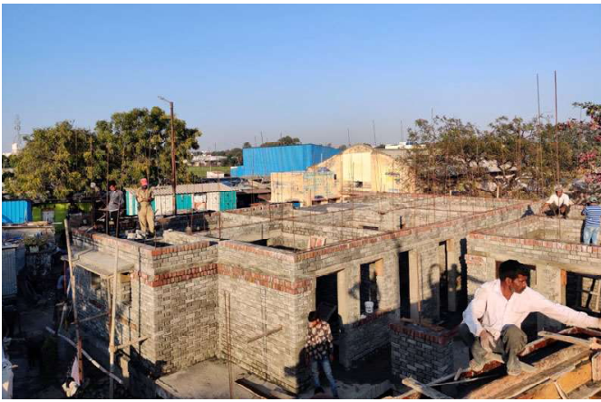
More photos from the construction of Building number 6, taken in September and October 2020. The black-cotton soil conditions on the site meant that the pile foundations had to go down five meters, so the foundations accounted for nearly 30% of the construction costs.
