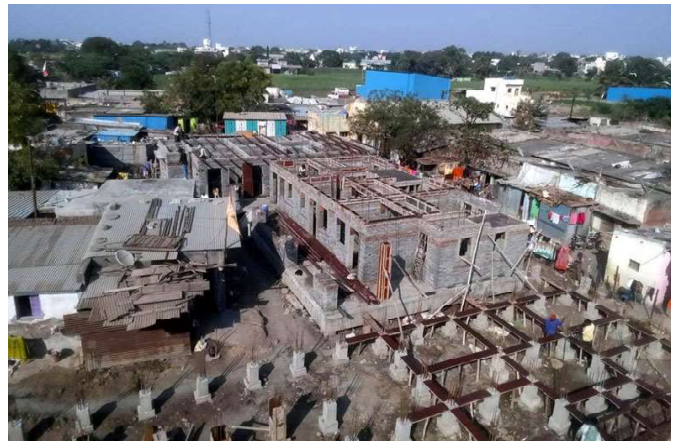
More photos from the construction of Building number 6, taken in September and October 2020. The black-cotton soil conditions on the site meant that the pile foundations had to go down five meters, so the foundations accounted for nearly 30% of the construction costs.
