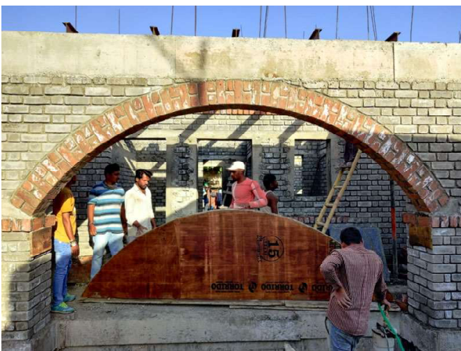
Here the arched walkways that will connect all the buildings are being constructed by the local contractor's masons on the site.
