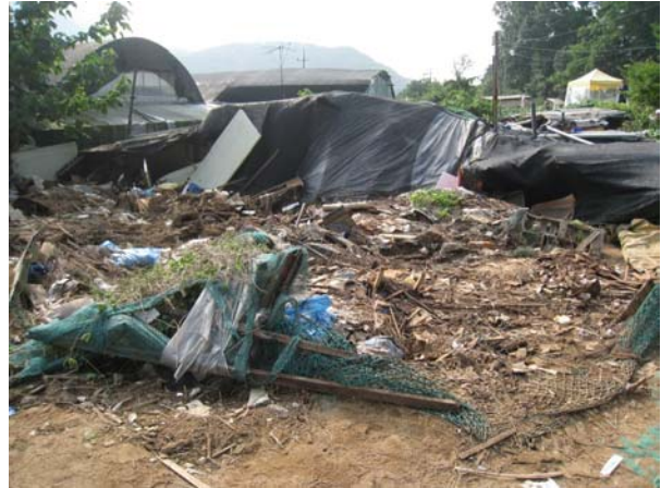
A resident's house was badly damaged by the landslide.
