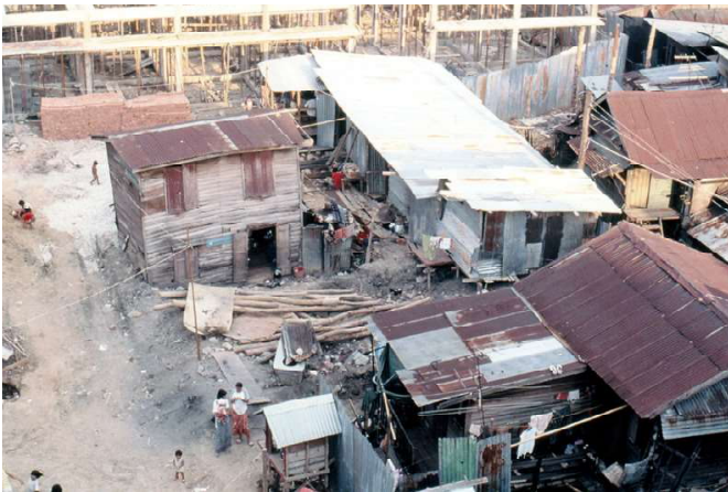
By 1984, construction of the concrete building frames had begun, at the back of the site, and people stayed in temporary housing in the front.
