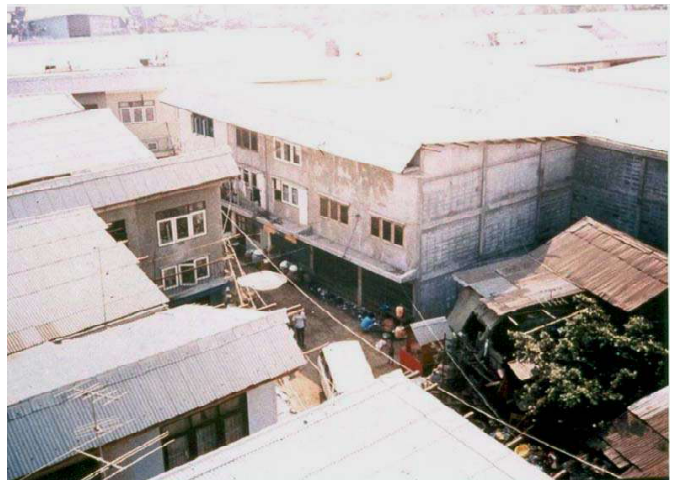
▲ A photo from 1985, when construction of the new houses was well along. To save money, the "core" houses were built by a local contractor, and then the families did the finish work themselves.
