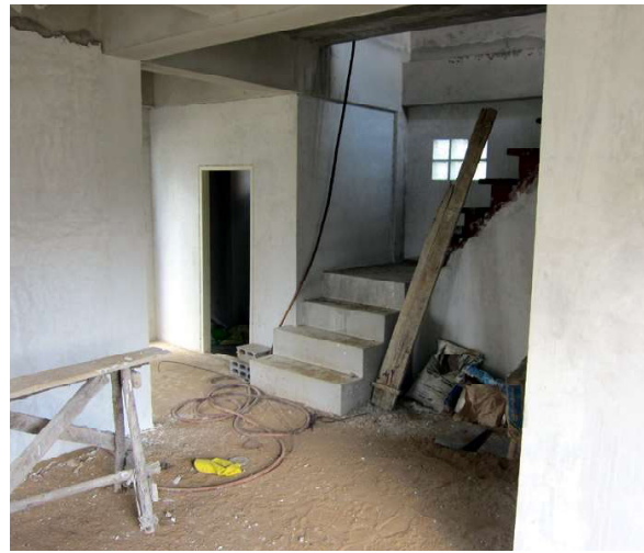
▲ The construction of the houses was not done by a commercial contractor, but by one of the network's "Community Builder" teams.
