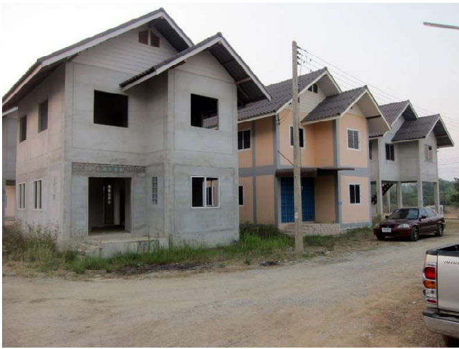
▲ Here are three almost-finished two-story houses. In the two on the left, the families have already enclosed the open ground floor space.
