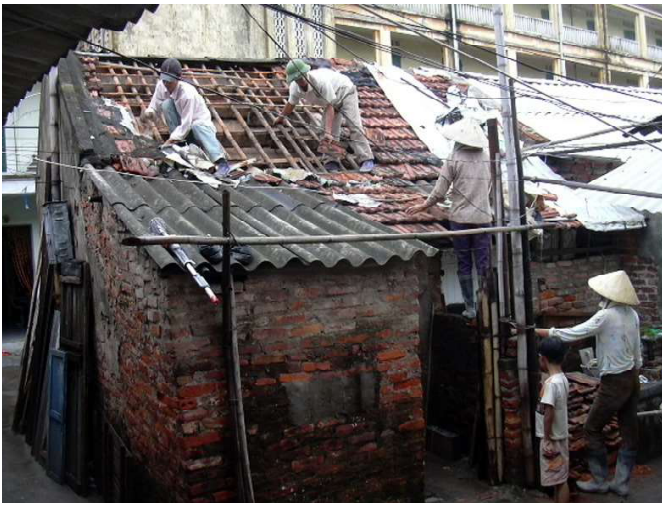
▲ The first step in the redevelopment was to dismantle the five middle houses to make way for the new central lane and drainage system.
