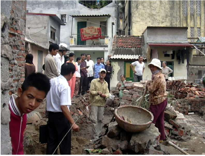
▲ The new houses were all built in batches of three or four, and here the first batch of houses are being marked out with string, to start the work of building the foundations.
