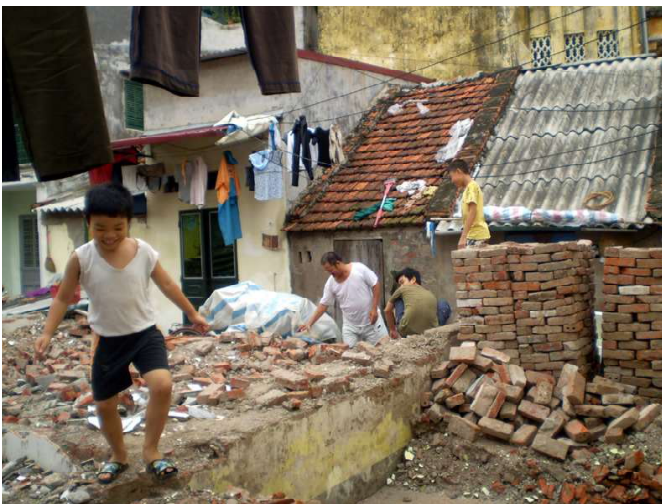
▲ Construction materials from the old houses (doors and windows, timber, bricks and roof-tiles) were carefully rescued and kept for using in the new houses, to reduce materials costs.
