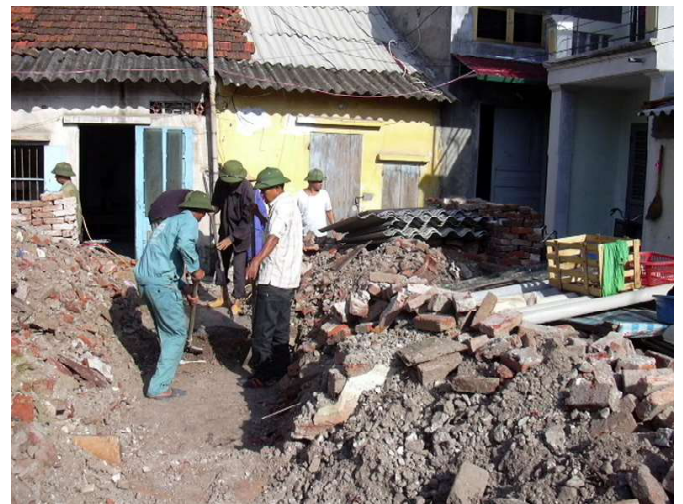
▲ Work starts on digging ditches for the new storm drainage system and piling up rubble to underlay the new, higher-up central lane, which would then be above the local flood levels.
