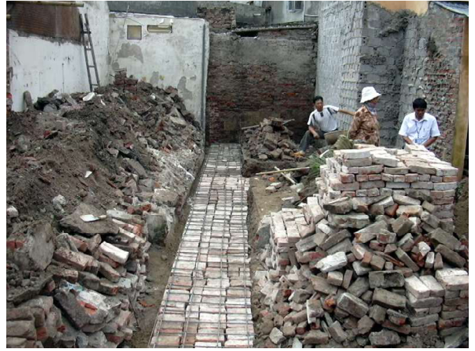
▲ All the the bricks salvaged from the old houses were put to use in laying the strong foundations for the new houses.
