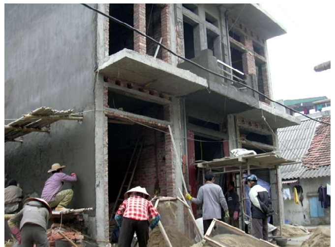
▲ It took less than three months to finish these first three houses, which tower over the old houses, which now look even sadder than ever.
