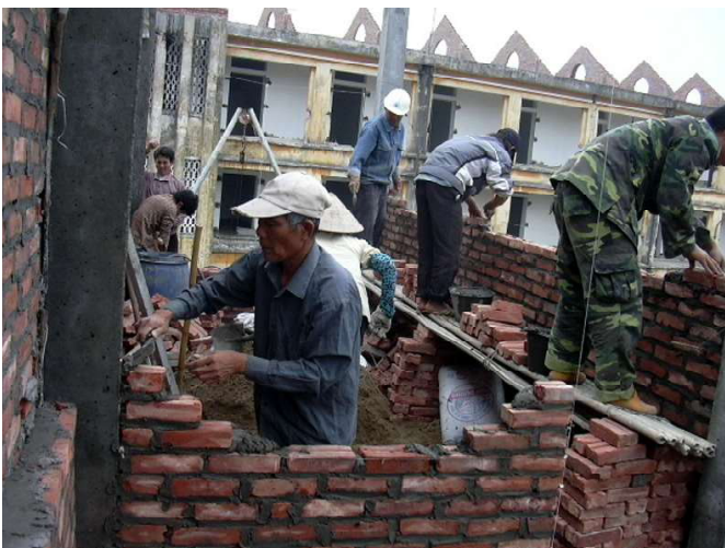
▲ The project unlocked so much energy and resources in the community, and the construction work progressed very fast.
