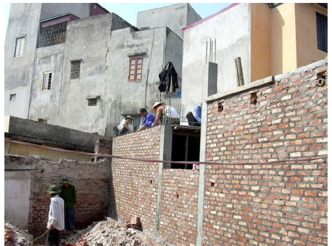
▲ Here some walls in the first three houses are going up. All of the houses used the standard building system of reinforced concrete frames and infill walls of fired bricks.
