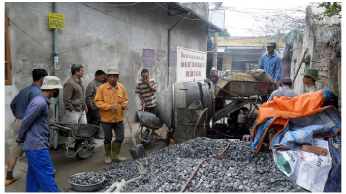
▲ Since it wasn't possible to bring trucks into the community, the sand, cement, gravel and other building materials had to be unloaded at the mouth of the lane, on Chi Lang Street, and then carried in by wheelbarrows. That's where the people set up the concrete mixing machine too.
