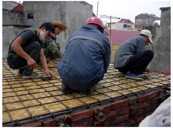
▲ Here some woven bamboo mats are being used as a base for laying the reinforced concrete floor slabs - an innovative and cost-saving technique.
