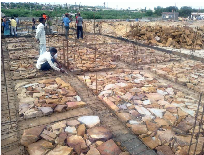
Work going on to lay the foundations for the heavy, load-bearing walls, which used blocks of local sandstone. The steel reinforcing at the corners is for seismic safety purposes.
