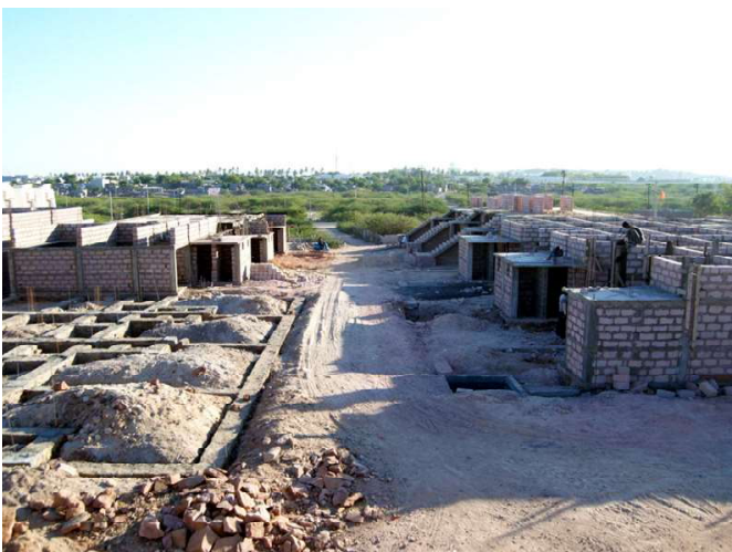
A photo of one of the sites where the construction is well along. Some houses are almost up to roof level and some are starting on the walls.
