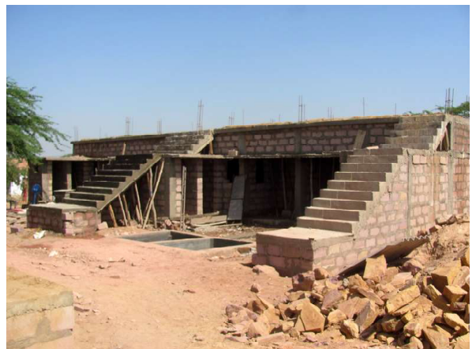
In this cluster of houses in Ramdev Nagar, you can see the underground tanks in the courtyard that will be used for storing water.
