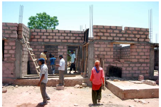
Here the walls are going up, with seismic reinforcing at the corners and in horizontal bands. The pinkish sandstone blocks are machine cut and come from quarry that is just fifteen kilometers away.
