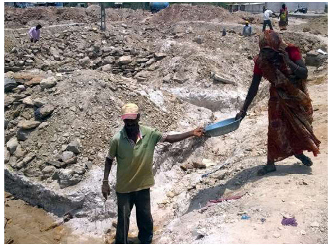
Digging the trenches for the foundations in the fierce Bhuj sun was hard work, but most of the families did it themselves, to save labor costs.
