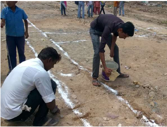
After the surveying team had pegged the house plots, the guidelines for digging the foundations were marked with lime powder.
