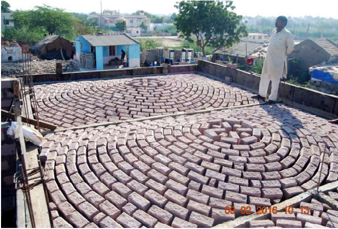
These shallow-dome roofs, made from the local sandstone, can carry the weight of concrete floor, without the need for any steel reinforcing.
