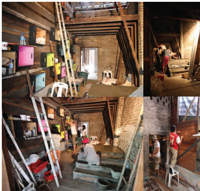
Changing the old house into a community library
