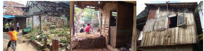
Flood impact: housing weathering & senimentation of solid waste
