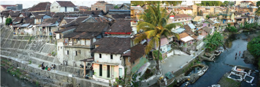
Upgrading project in Kampung Kali Cho-de, Yogyakarta, Indonesia
