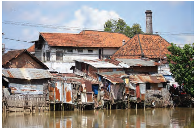
Typical look before renovation
