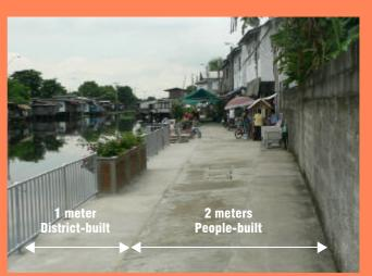
Here is a section of the newly-completed canal-side lane, with the inner 2-meters built by the community (with main drainage lines underneath) and the outer 1 meter part built by the District, on land reclaimed from the canal, with the railings, planters and steps down to the canal.
