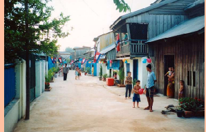
AFTER UPGRADING : And here is a photo after the underground drains have been laid, the road completely concrete paved and the houses have been repainted and decorated with small planting strips for flowers and trees.
