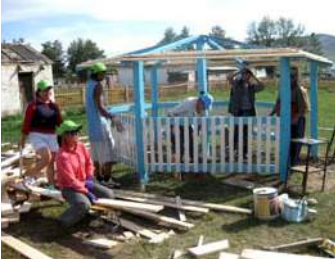
▲ A cheerfully-painted gazebo being built by community people in one of the ger areas in Erdenet. Land isn't the problem in these ger areas, but access to basic services and infrastructure is.
