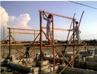
▲ Constructing new "starter" houses in a portion of the sprawling Baseco slum in Manila, after a fire destroyed the area.
