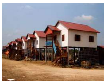
Before and After : The old riverside Monorom slum in Serey Sophoan, and the new houses on free government land.
