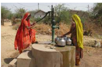
▲ The new hand-pump and concrete apron at Bapa Diyal Nagar slum, in Bhuj.
