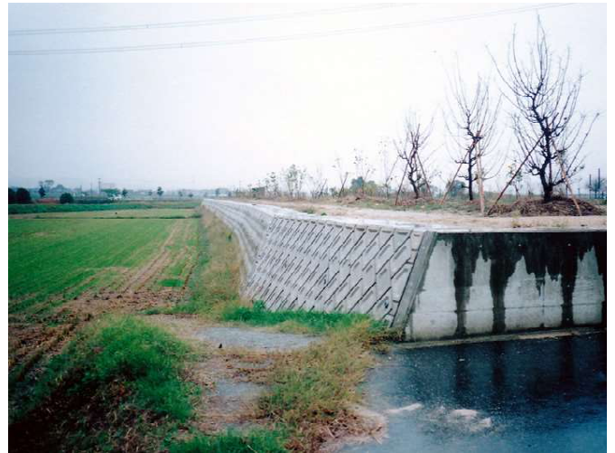
The embankment built along the Homan River stopped the flooding and allowed the community to reclaim more land for their housing and other community amenities.
