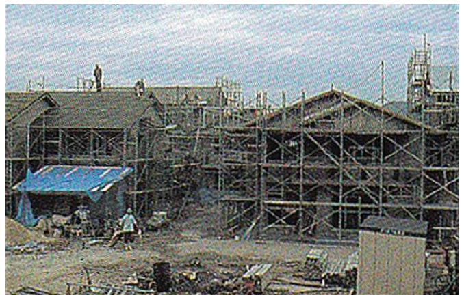
Here the public rental housing is being built in the center of the newly-redeveloped Misaki. The local government hired contractors to build the housing, but following the people's designs.
