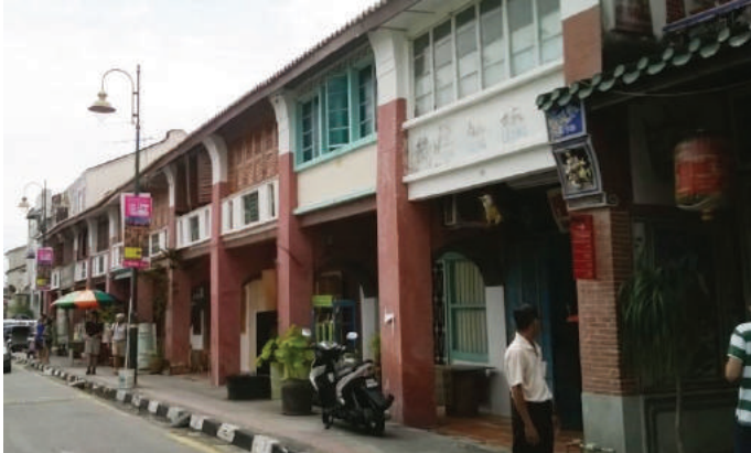
Before and after façade treatment.
