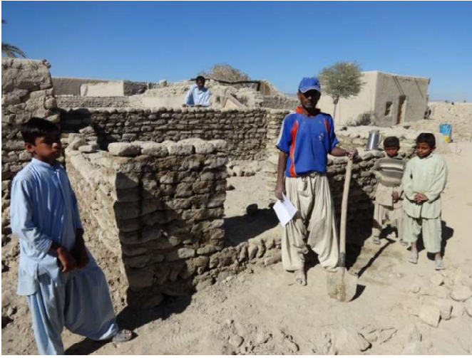
Here one of the heavier, thicker walls is being constructed, using some mud blocks salvaged from the rubble and some newly-made on the site by the mason.
