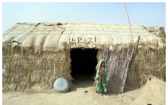
This is another house type that was built by families who could not afford a mud-walled house yet but urgently needed shelter. In this system, palms and palm thatch are tied to bamboo frames to make quick, light and well-insulated walls.
