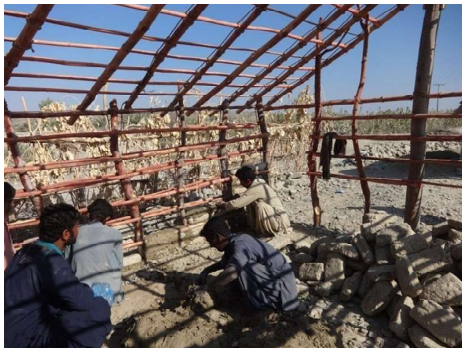
These two photos show one of the roofing systems the people in Awaran used to rebuild their houses after the quake. This was one of the quicker and lighter systems, in which mud and mud blocks (both newly-made and salvaged from the rubble of their old houses) are packed around a reinforcing framework of treated bamboo poles tied together with rope.
