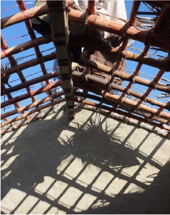
The first step in roof building is to erect a criss-crossing framework of treated bamboo poles, of varying thickness, tied together with rope.
