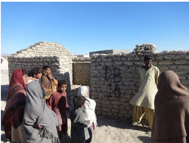
Here is a thick-walled house made of mud blocks all ready for the final plastering, before the new roof is put on.
