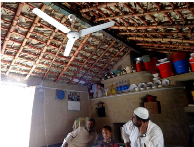
Inside one of the completed houses, in which you can see the beautiful pattern of overlapping "peesh" palms in the roof above the bamboos.
