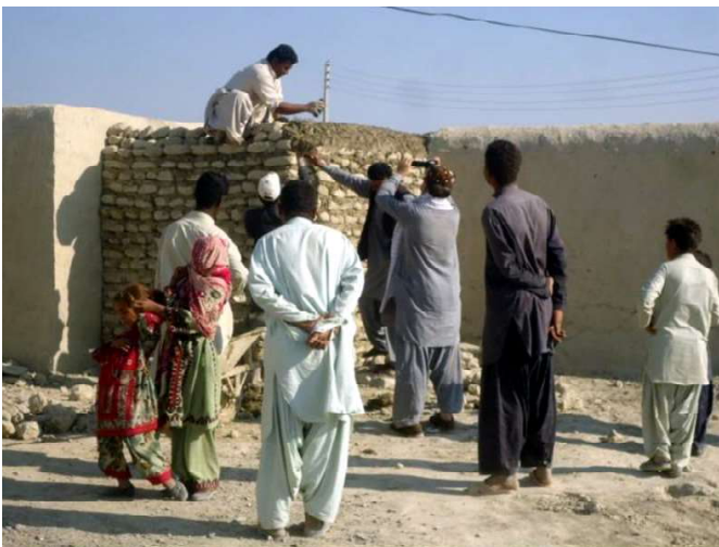
A bathroom being built onto the back side of a house, using the thick-wall system, with mud blocks and fiber reinforced mud mortar.
