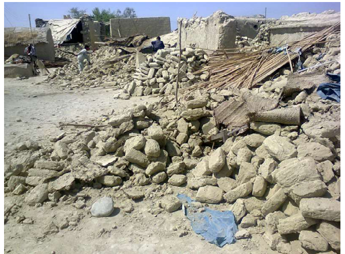
In this photo, you can see where families have begun to make piles of useable adobe blocks and other building materials salvaged from the rubble.
