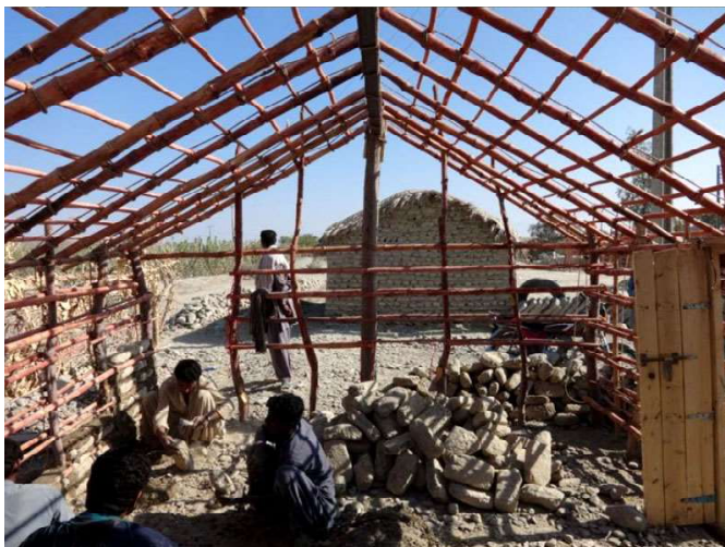
These two photos show one of the roofing systems the people in Awaran used to rebuild their houses after the quake. This was one of the quicker and lighter systems, in which mud and mud blocks (both newly-made and salvaged from the rubble of their old houses) are packed around a reinforcing framework of treated bamboo poles tied together with rope.
