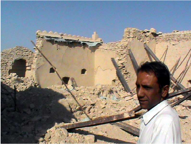
The people build their houses from materials available locally, like stone, mud and a little timber for the roofs, doors and windows. Many were killed by heavy flat roofs collapsing and crushing the people inside the houses.
