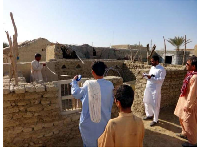
Another thick mud-block wall going up, reinforced by vertical timbers and using a wooden window salvaged from the old house. You can see some ornamental niches set into the back wall.
