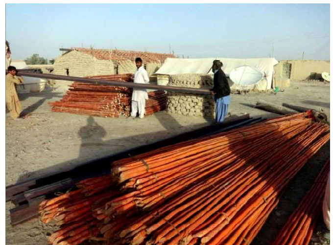
These are the treated bamboo poles, in various thicknesses, that will be used for both the roofs and some of the walls.
