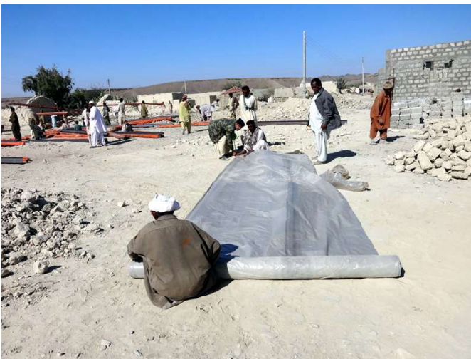
Some families added a layer of this plastic sheeting on top of their roofs, to make them even more waterproof. But the gusty winds made it hard to put the material up, and many families decided not to use it.
