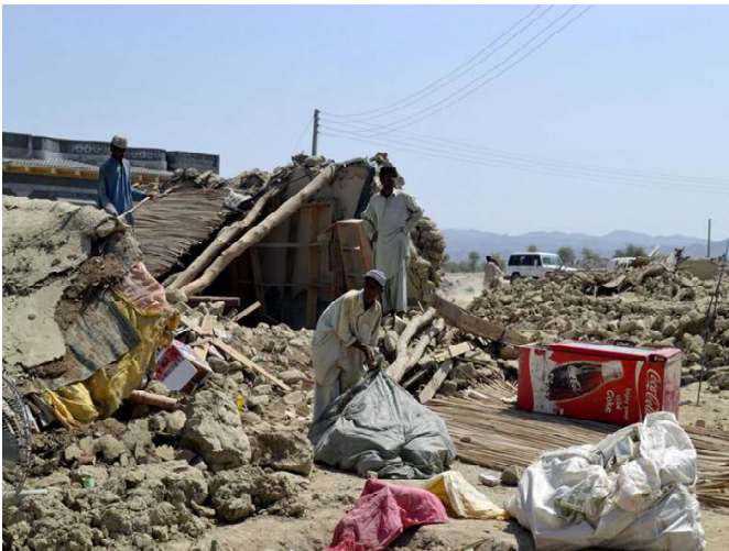
When the URC team first came, they found many families still sifting through the rubble to find useable materials for rebuilding their houses.
