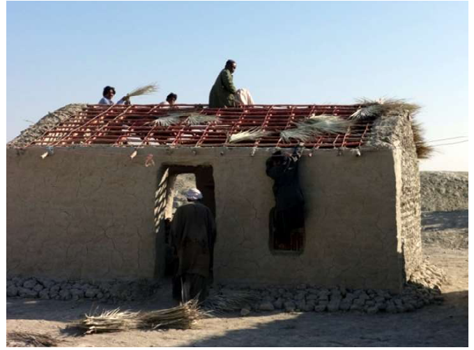
The first layer of roofing is made of "peesh" wild palm leaves that are tied to the bamboo frame in decorative overlapping patterns that can be seen and admired from the room below.
