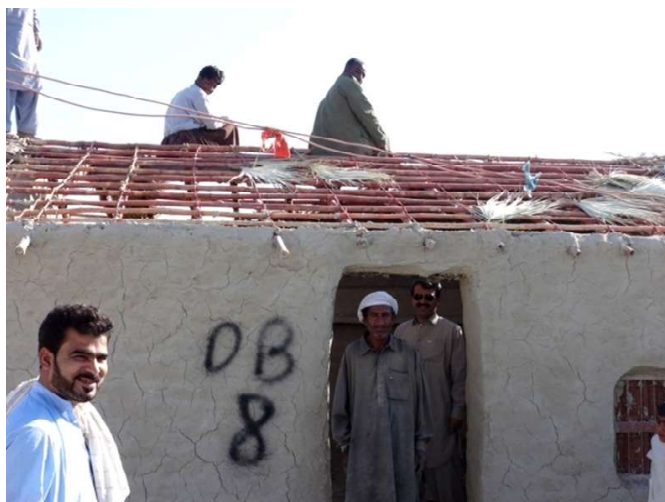
Here the walls have been plastered with mud mixed with wheat straw or grass fibers, to make it harder, more stable and more waterproof.
