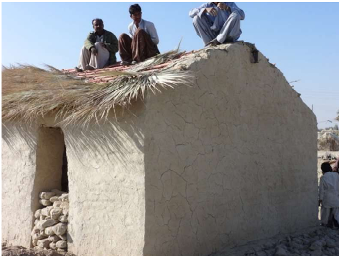
The wild palms are tied in such a way as to create an overhang along all four edges of the roof, to prevent rain from dripping down the mud walls.
