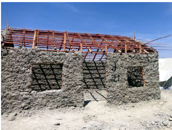
Here the bamboo-reinforced mud block walls have been completed and are ready to be plastered inside and out with mud.
