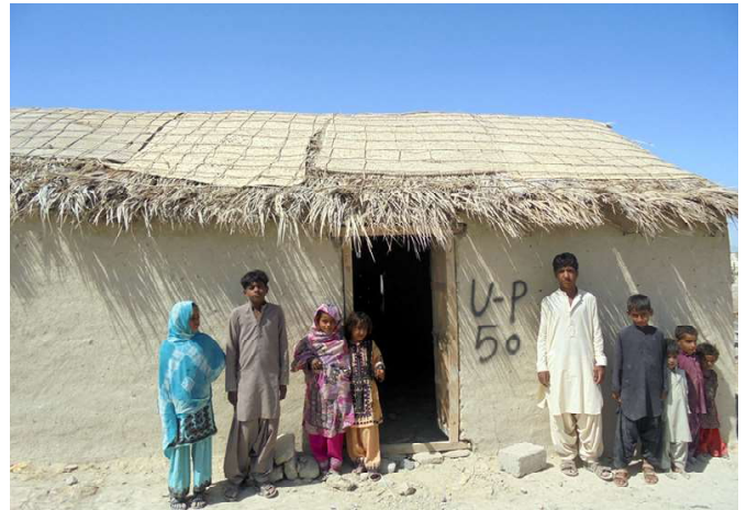
On top of the wild palms, tightly woven palm mats are tied down with stout rope to keep everything in place in the fierce Awaran winds. Some families added a layer of plastic sheets on top, but for most, this is the completed roof.
