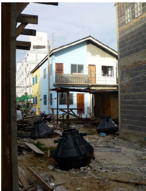
▲ The construction process was tightly organized, with committees in charge of various aspects of the project, and the building work went quickly.
