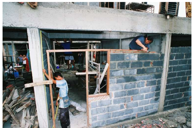
▲ The community members did all the construction themselves, working in teams to construct the houses together, in batches.
