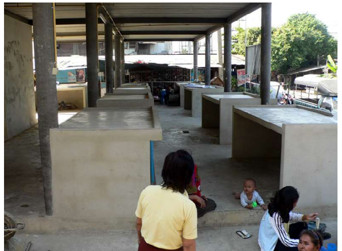
▲ This is the community's own market, just after the construction was wrapping up in 2005.
