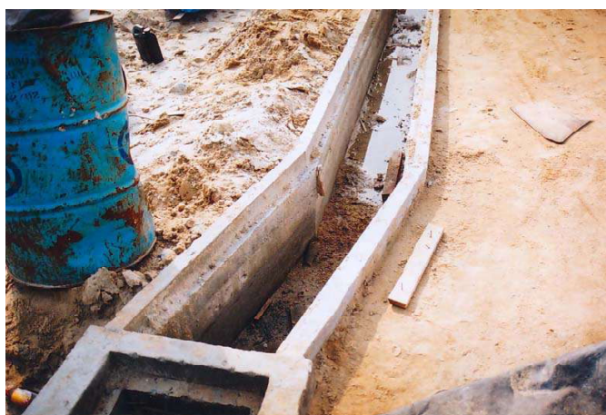
Making the storm drains and pile foundations was very difficult and expensive, because of the thick concrete that had to be drilled through.
