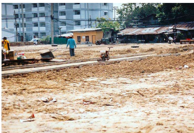
The resettlement site was covered with a thick layer of reinforced concrete, but still needed 80 cm of soil on top to bring it above flood level.
