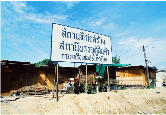
▲ As soon as the relocation deal was struck, the Port put up this sign announcing the construction of a container storage facility on the Block 7-12 site.
