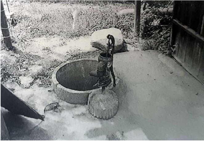
There was no piped municipal water in the settlement, so people had to pump water for washing and cooking from a few open wells like this.
