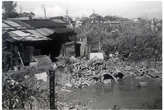
Some 200 of the houses were built right in the Yamoto riverbed, and got flooded almost every year during typhoon season.
