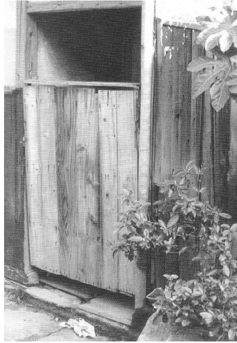
There were no sewers either, so the 900 families had to make do by sharing a few pit latrines like this one, here and there in the community.
