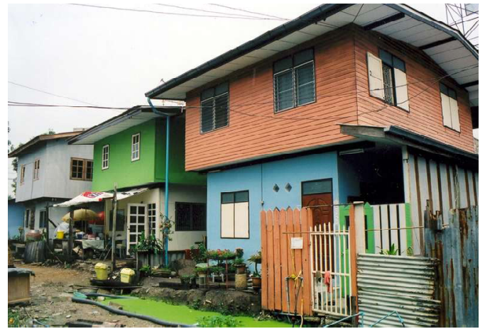
Another photo showing how the construction of the new houses went on while the roads and infrastructure were still underway.
