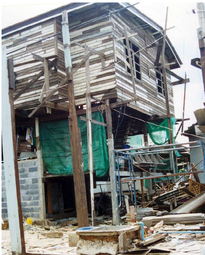
▲ This family decided to renovate their old wooden house and lift it up on tall concrete stilts, so a new ground floor could be built underneath.
