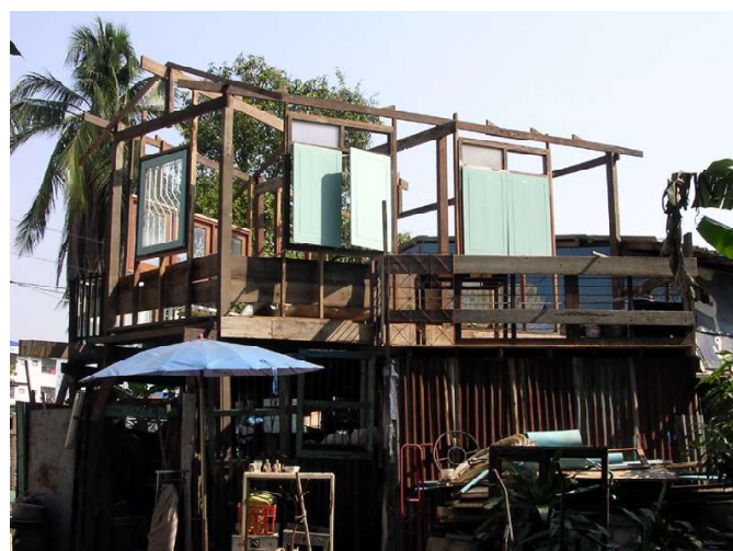
▲ To save money, many families carefully dismantled their old wooden houses and used doors, windows and timber in their new ones.
