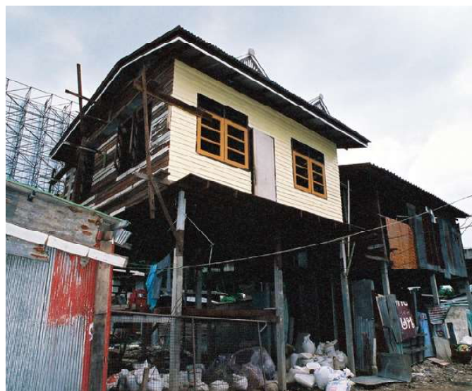
▲ This family decided to renovate their old wooden house and lift it up on tall concrete stilts, so a new ground floor could be built underneath.
