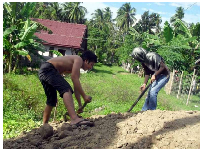
There were patches of stagnant water in low-lying places in the community, and these had to be filled in before construction could start. Once the trucks dumped the infill soil, it had to be spread out. Some of this work was done by machines loaned by the municipality, and some had to be done by hand, with shovels.
