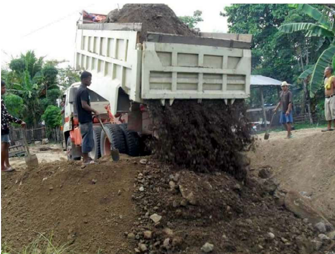
There were patches of stagnant water in low-lying places in the community, and these had to be filled in before construction could start. Once the trucks dumped the infill soil, it had to be spread out. Some of this work was done by machines loaned by the municipality, and some had to be done by hand, with shovels.
