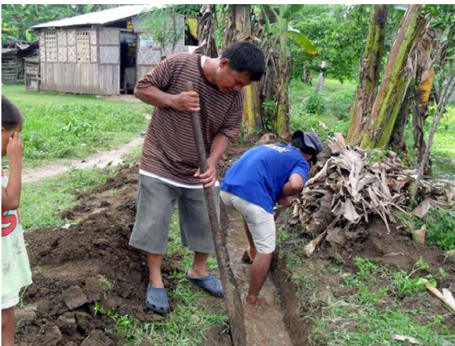
Here the difficult work is going on to dig new trenches which will divert the water from the creek away from the house plots. On the right, the new ditch, ready for concreting later.
