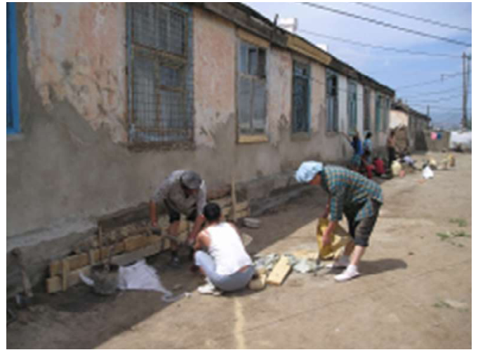
The fierce, snowy Mongolian winters take a big toll on buildings, and the outside of the Yaarmag barracks had crumbling plaster and broken window and door frames (above left). The photo on the right shows the work going on to repair the facades, before repainting.
