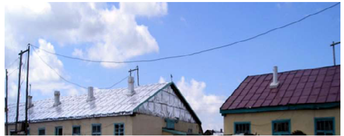
These photos show the work going on to remove the old, leaky asphalt roofing shingles (above left), which were replaced with insulated and water-tight interlocking galvanized iron sheets (above right).
