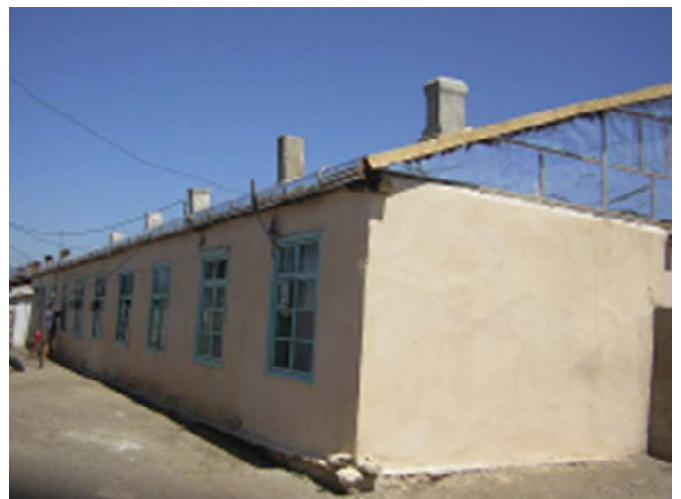
Two photos which show the finished work on the facades, with re-plastered walls, repaired foundations, repaired windows and door frames and a new coat of pale yellow for the walls and a cheerful cornflower blue for the window frames.
