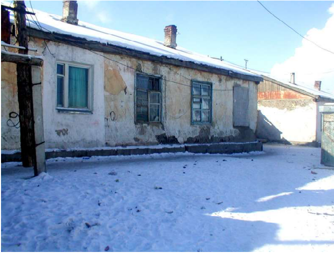
These photos show the Yaarmag barracks buildings, in the winter, before the upgrading project began. Services like water supply and toilets were primitive, and the buildings were in bad repair, with crumbling walls, leaky roofs and lack of proper drainage.
