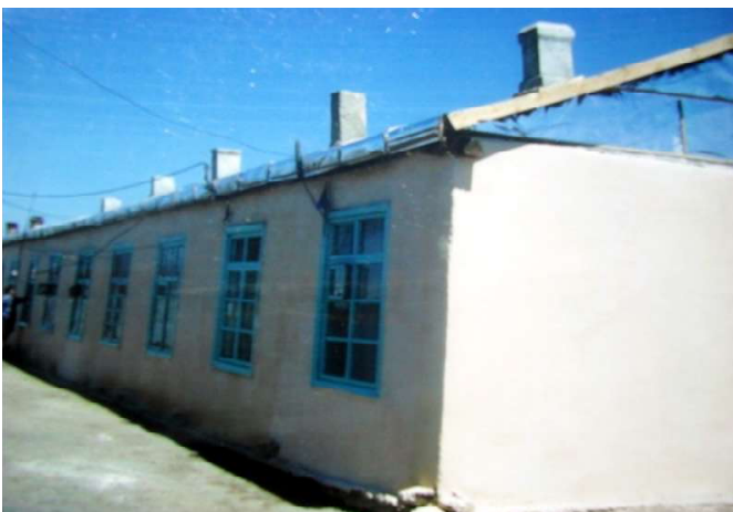
Two photos which show the finished work on the facades, with re-plastered walls, repaired foundations, repaired windows and door frames and a new coat of pale yellow for the walls and a cheerful cornflower blue for the window frames.
