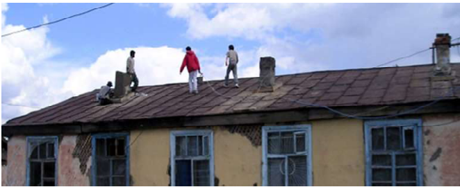
These photos show the work going on to remove the old, leaky asphalt roofing shingles (above left), which were replaced with insulated and water-tight interlocking galvanized iron sheets (above right).
