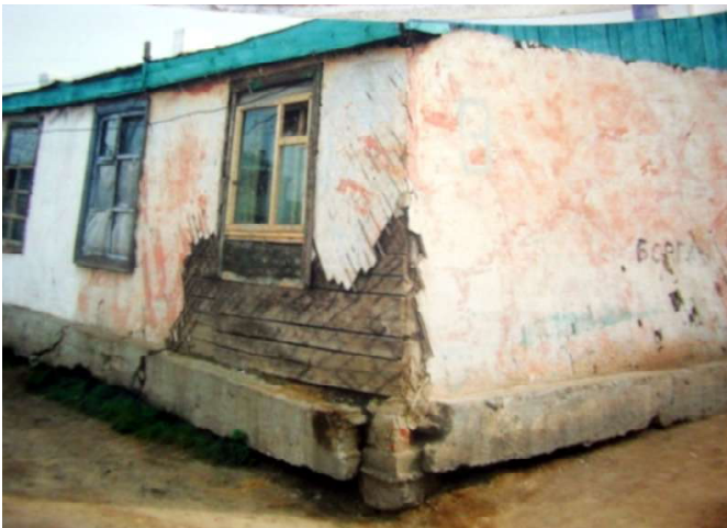
The fierce, snowy Mongolian winters take a big toll on buildings, and the outside of the Yaarmag barracks had crumbling plaster and broken window and door frames (above left). The photo on the right shows the work going on to repair the facades, before repainting.
