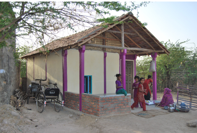
Photograph 45 . Diaben's completed home.
