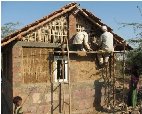
Photograph 41 . Construction process, alternate technologies of building were employed
